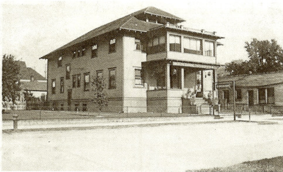
Bronson Hospital before remodeling - 1925
