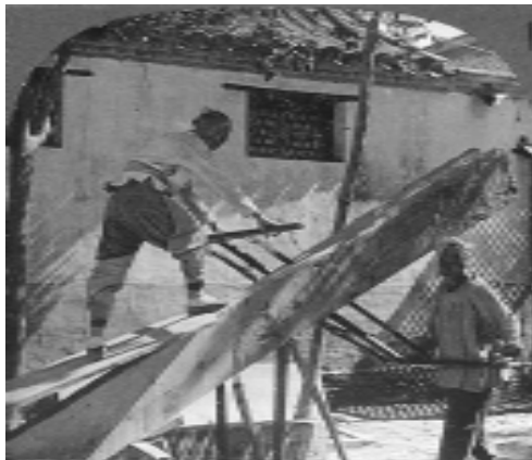
The Chinese laborers who came to America were hard workers who did the down and dirty jobs no one else would do. Above two workers hand-cut a beam using a pit saw.
